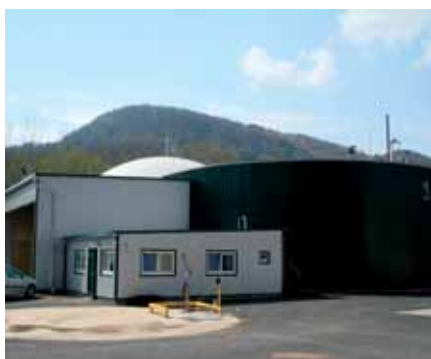
Bio Energie Anlage
